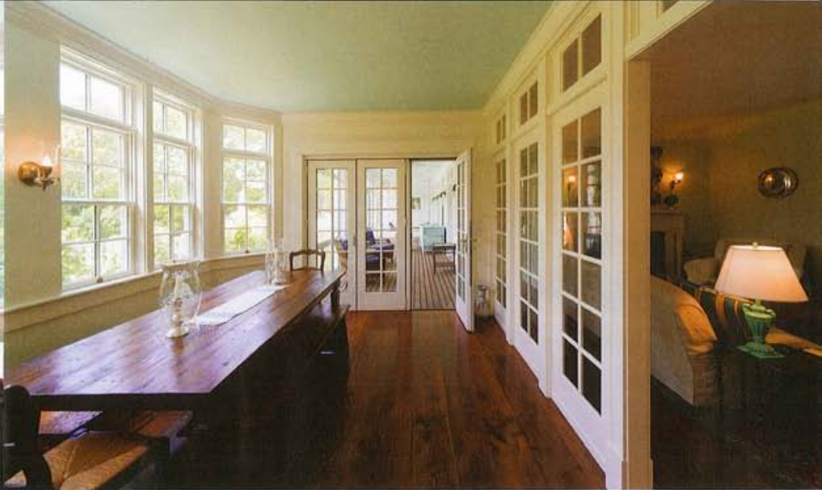
The house reconstruction included creating a glass wall between the dining and living areas to allow more natural light into the interior.
